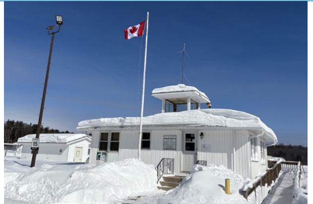
Terminal Building Airport Facility
